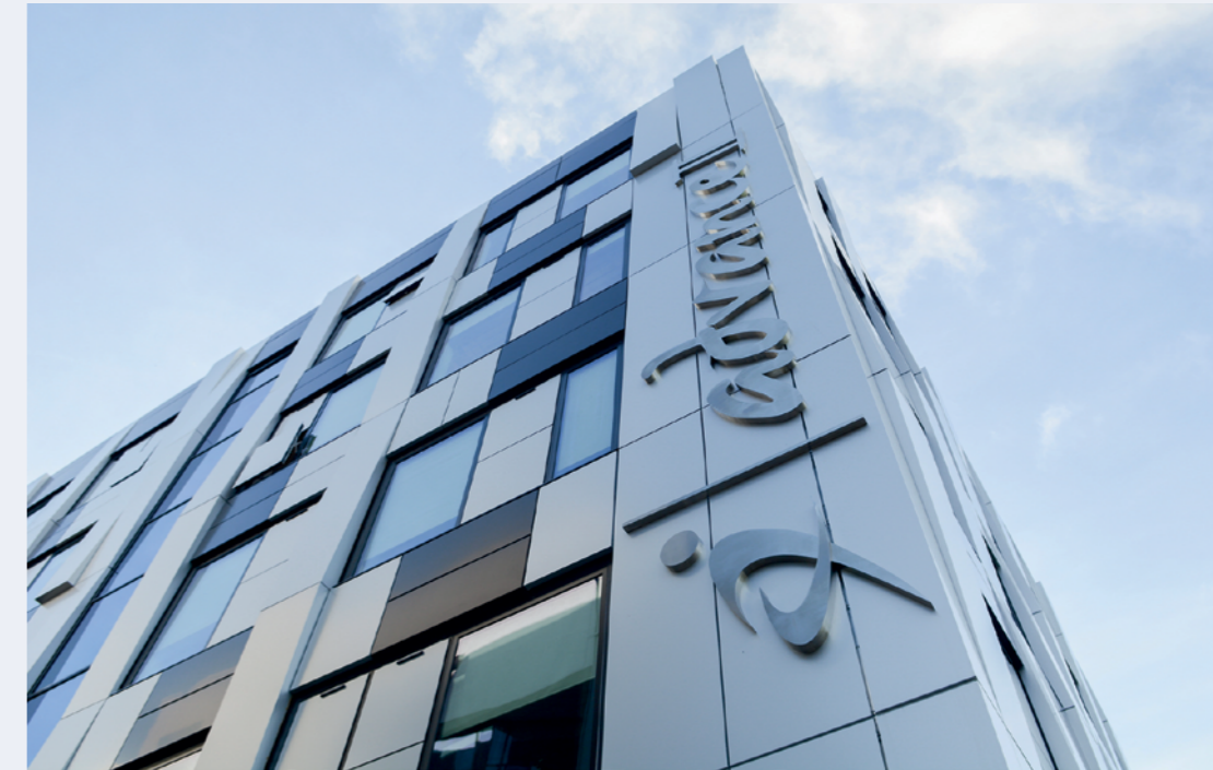
FIGURE 06 Insurance-Backed Alliancing pilot project, Dudley College Advance 2 building, 2017. Photos IPInitiatives.
